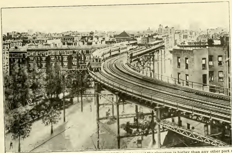
ELEVATED RAILWAY CURVE AT 110TH STREET —At this point the elevation is higher than any other part of the city, reaching a height equal to five stories and requiring elevators at the station to take up and down the passengers. New York City is famous for its elevated Railroads, this being one of the most noted sections.
